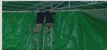
Fitting on and securing the flexible liners
