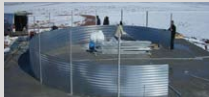
Completion of the first ring
