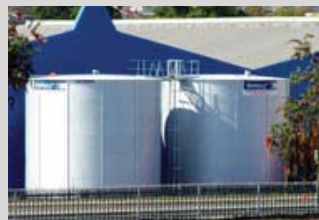
Industrial water supply
