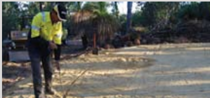
Marking out the tank diameter
