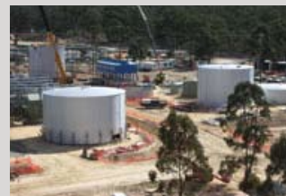
Water supply for mining
