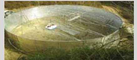
Fitting on the dome truss
